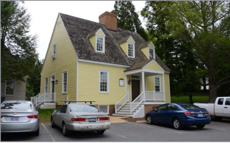
Jefferson's birthplace house replica, ca. 1960, was removed from Shadwell Plantation, and is now located in a colonial-style office park outside of Charlottesville, where it serves, at the moment, as the office of a collegiate sports media rights management company. CLUI photo
