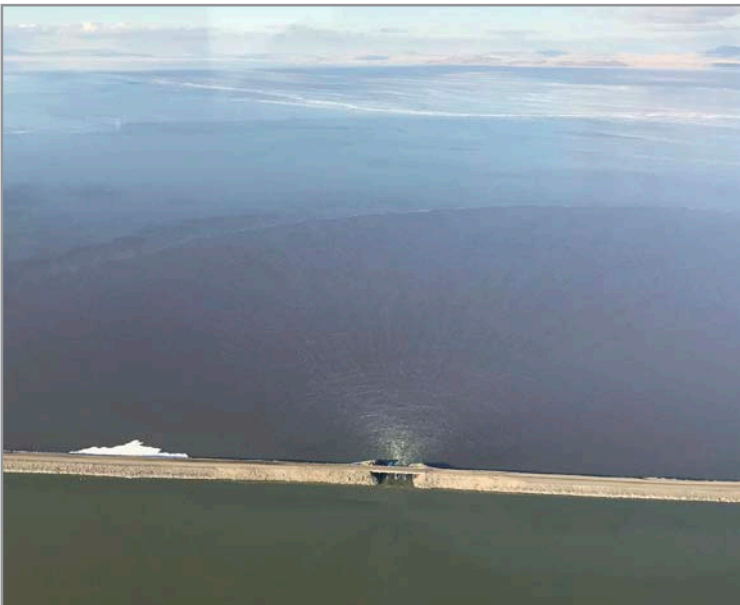
The south half of the lake, three feet higher than the north half, flowing through the new breach in the causeway. CLUI Photo by Hikmet Sidney Loe
