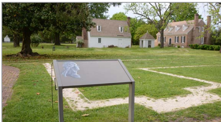
The footprint of George Washington's birthplace home at Wakefield is sketched in a white outline, like chalk around a body at a historic home crime scene. An inaccurate replica of the house, constructed in the 1930s, on the wrong foundation, is in the background. CLUI photo
