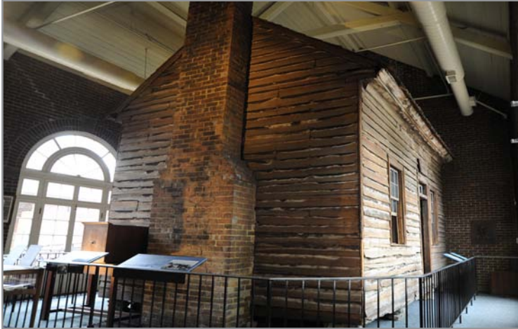
Andrew Johnson's tailor shop in Greenville is inside a structure built around it by the state in 1923, and purchased by the National Park Service in 1963. CLUI photo
