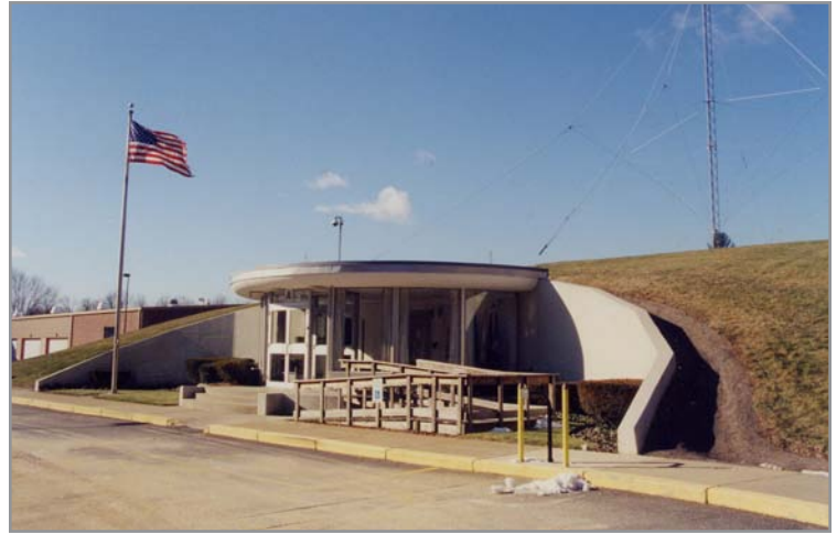
The Federal Emergency Management Agency's regional operations center for New England is housed in this underground bunker in Maynard, outside Boston. Built in the early 1960s, when the agency was more concerned about nuclear attacks than it is now, the bunker has an operations room for organizing emergency relief teams throughout six New England states, and a variety of communications antennas on the roof of the building. CLUI photo
