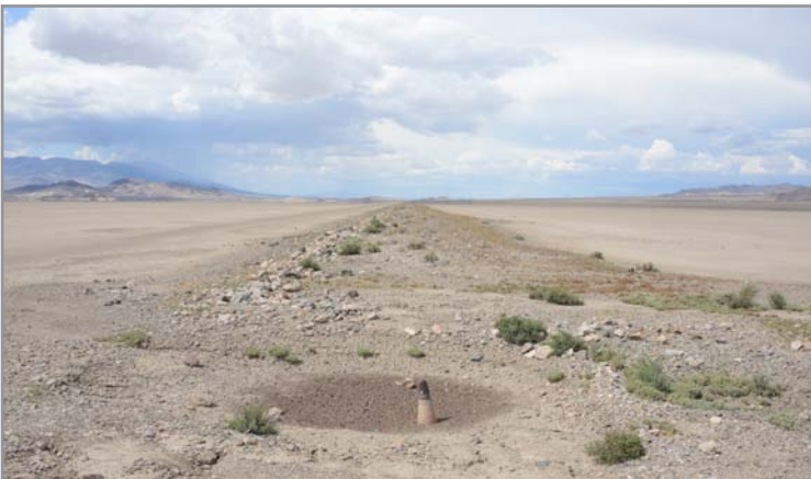
View down old railroad roadbed running through Silver Lake, Nevada. Dry lakes often are the path of least resistance for power lines and railways. CLUI photo
