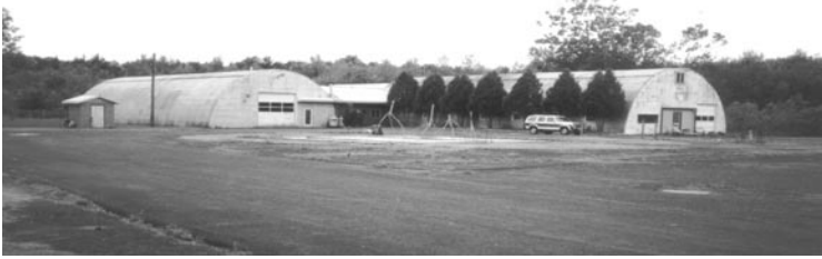
Quonset huts at the missile silo site that has been refurbished by Art Works, near Plattsburg, NY. Michael Kassner photo
