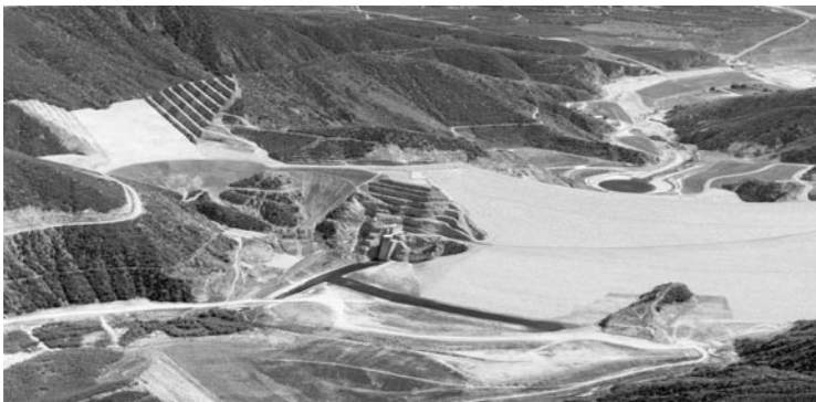
Seven Oaks Dam, a flood control structure in the San Bernardino Mountains, is a $420 million earthmoving project, completed just a few years ago. CLUI photo
