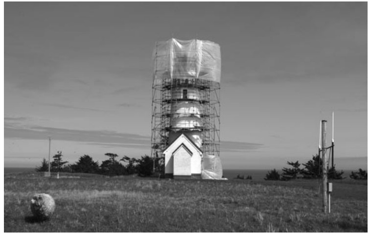
Cape Blanco lighthouse, being restored.
