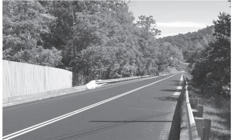
Travellers on the highway have no clues that they are driving over the top of natural bridge when they approach the community of Natural Bridge. The bridge has had a road on it for over 150 years. CLUI photo
