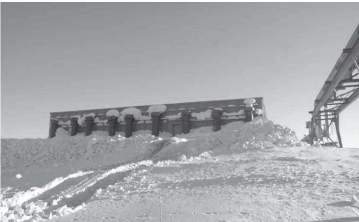
The buildings are connected by steampipes, and vented underneath, so that the heated buildings do not melt the permafrost. CLUI photo
