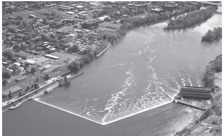
The first full obstruction on the Hudson River from Manhattan is the Federal Dam. This marks the end of the river as a tidal estuary, 150 miles from Battery Park. A lock on the east side of the dam allows boats to continue northward, and through a long series of locks, into the Great Lakes via the Mohawk River and Erie Canal, and to the St. Lawrence River in Canada, via the Champlain Canal. CLUI photo
