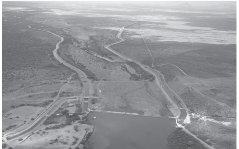
Located on the Salt River, just below the confluence of the Verde River, the Granite Reef Dam is the main distribution point for the water that supplies Phoenix. Several canals intersect or originate here, upstream of the city. CLUI photo
