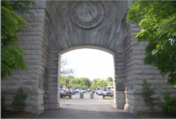
The façade of the main entry of the Adams Power Plant was moved to Goat Island, to form a gateway into the park's concession area. CLUI photo
