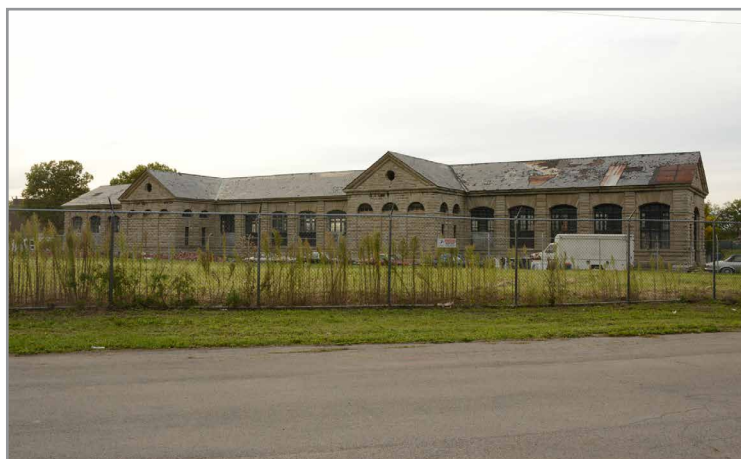
The transformer building, designed by McKim, Mead and White, is the only remaining structure from the Adams plant. Though it is in disrepair, there is talk of turning it into a museum about the site's important hydropower history. CLUI photo
