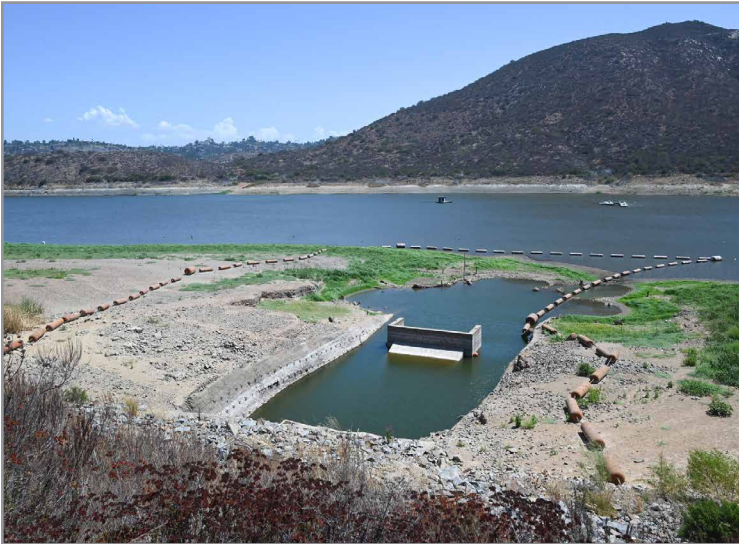
Intake/outfall for the pumped storage plant at Lake Hodges, in San Diego County. CLUI photo
