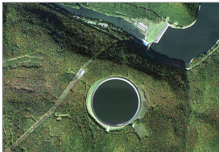
The upper reservoir of the Seneca Pumped Storage Project is perfectly round, 2,500 feet across, and 800 feet above the Allegheny River. Google Earth image
