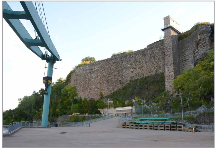
The remains of the Schoellkopf Power Station at the base of the gorge were removed in 1962, when the area was cleaned up during the third wave of hydroelectric transformation at Niagara Falls. Today the power station site is accessed by the old elevator shaft on the edge of the gorge (right), and is the winter home of the Maid of the Mist tour boats, which are picked out of the river with a giant crane (left). CLUI photo
