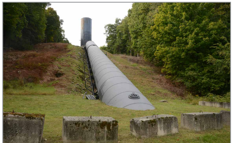
The penstock at Rocky River is a 1,000-foot-long, 15-foot-wide pipe that connects the plant to the reservoir, and is topped by a standpipe that allows water to escape during a surge in pressure. CLUI photo
