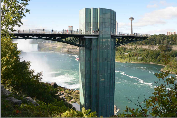
Like a dipstick displaying the hydraulic head between the top and the bottom of Niagara Falls, the Prospect Point Observation Tower is the penstock for the flow of tourism on the US side of the falls. Up to eight million visitors a year line up on the gangplank and stream through elevators to head into the soaking vapor on the Maid of the Mist boats, at the base of the tower. While tourists migrate towards the falls, local hydroelectric projects have been all about how to avoid them. CLUI photo
