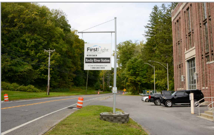
The Rocky River Station is easy to find, located on Highway 7, north of New Milford, Connecticut. It was built by the Connecticut Light and Power Company, and is now operated by FirstLight, a regional renewable energy company. CLUI photo
