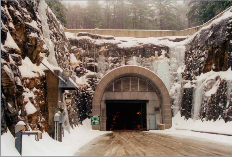
The powerhouse at Northfield Mountain is deep inside the mountain, and all the pipes and penstocks are underground too, bored through solid granite. CLUI photo
