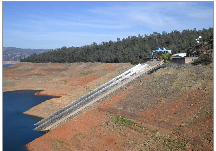
The intake pipes for the Edward Hyatt Power Plant at the Oroville Dam. The plant is one of two at the Oroville-Thermalito Complex that can pump water as well as produce electricity. CLUI photo
