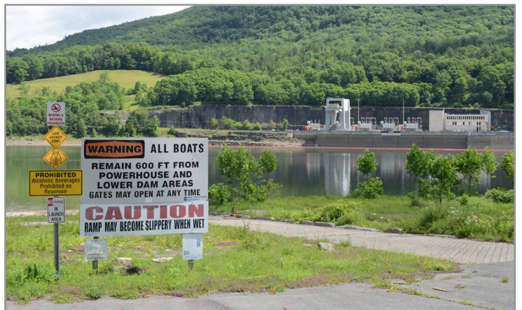
Blenheim-Gilboa's powerhouse is on the riverbank at the base of Brown Mountain, where its upper reservoir is located. There are four pump/turbines that both lift water to the upper reservoir and produce 1,100 megawatts of electricity when water flows back down through them. CLUI photo
