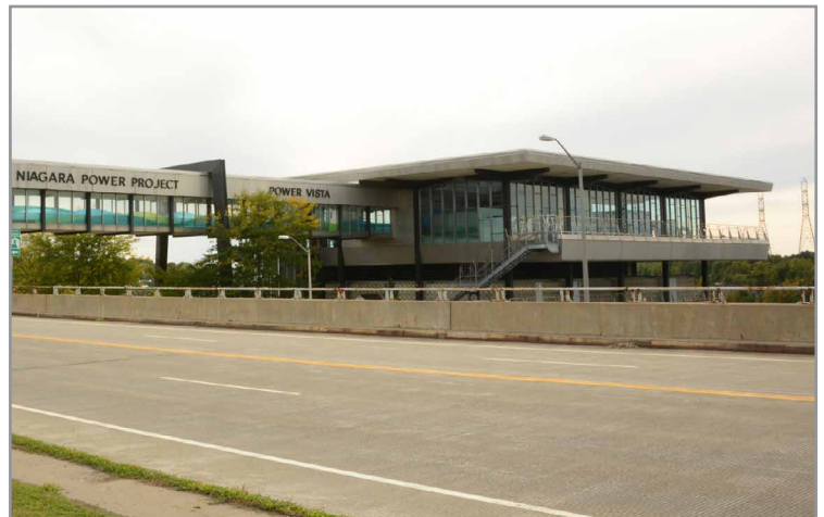
The Power Vista, accessed by a skybridge over the Robert Moses Parkway (also known as the Niagara Scenic Parkway), perched atop the gorge, with a view up and down the river, is the ne plus ultra of hydropower visitor centers in the USA. CLUI photo
