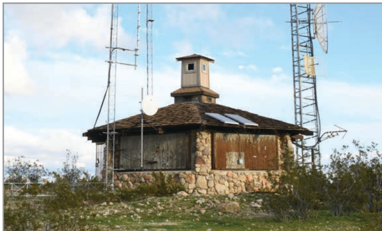
The former overlook pavilion atop Galileo Hill.
