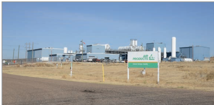
Air Products helium gas plant in Liberal, Kansas. Several non-critical elements exist in gaseous form, and are harvested in air separation plants, or, more commonly, manufactured at petrochemical plants, which are abundant in the US. CLUI photo
