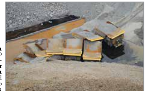
The Bingham pit landslide went from top to bottom of the 3,000 foot deep pit, forming a half mile-wide gash in the stepped slope. It took out part of an equipment maintenance building, and buried nine giant yellow dump trucks. CLUI photos
