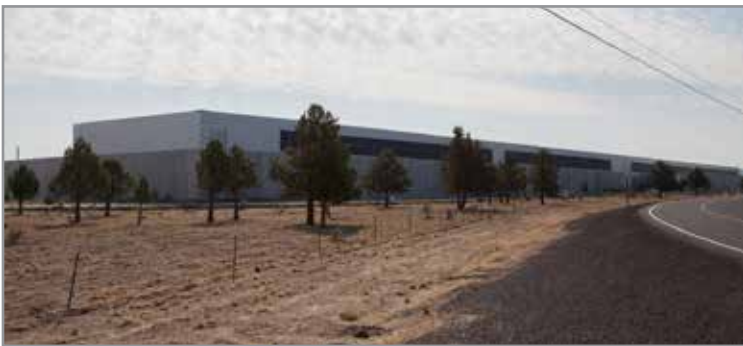
Facebook built its first company-owned dedicated data center in the remote central Oregon town of Prineville in 2010, and opened another one next to it in 2013. Apple operates a data center nearby. CLUI photo
