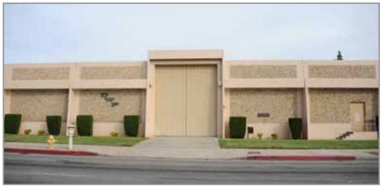
Distributing Station #88 in Chatsworth was built in 1973 in a sort of functional institutional modernism typical of the distributing stations of the San Fernando Valley. CLUI photo
