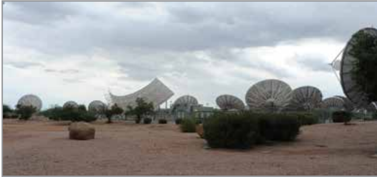
The Echostar satellite facility in Gilbert, Arizona, is one of the company's largest uplink sites. Echostar operates several earthstations in the USA for its network of communication satellites, serving video and data transmission customers. CLUI photo
