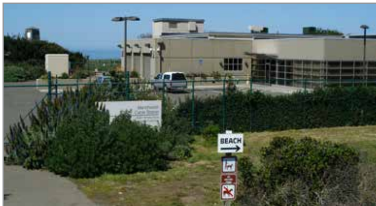
The Manchester Cable Station in Northern California is one of a few dozen trans-oceanic fiber optic cable landing stations along the East and West Coasts. CLUI photo
