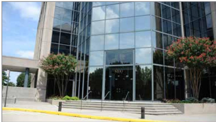
An office building at 8100 Boone Boulevard in Tysons Corner, Virginia, was the original Metropolitan Area Exchange for the eastern United States, with half the nation's internet traffic passing through it in the early 1990s. Today it is still a well-connected data center in the region of the Dulles Corridor, the highest concentration of internet infrastructure in the nation. CLUI photo
