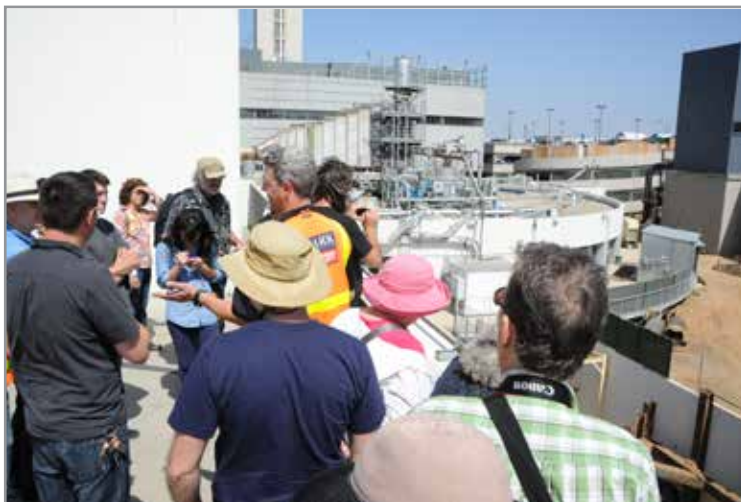
The group gets a briefing from a Clark/McCarthy engineer working on the Central Utility Plant upgrade in the heart of LAX. CLUI photo
