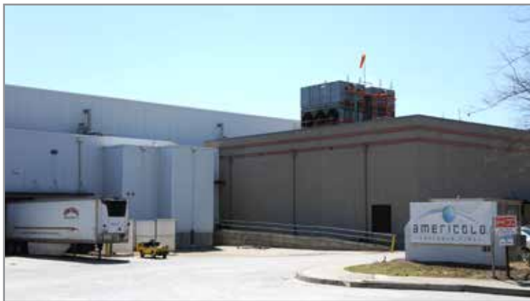
An Americold cold storage warehouse outside Atlanta, Georgia, with a reefer trailer from Central Refrigerated, of Salt Lake City, and the tell-tale orange windsock that all refrigerated warehouses have, to indicate wind direction in case of an accidental release of the refrigerant, ammonia. CLUI photo
