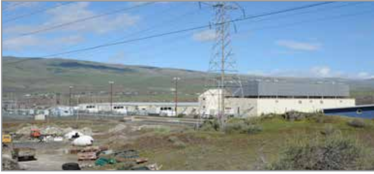
Google built its first dedicated data center outside Silicon Valley in The Dalles, Oregon, in 2006. It cost around $600 million. There are now three buildings on the site. It is located across the street from the site of a former aluminum plant. The aluminum industry once flourished along the Columbia, using power from the dams to produce the metal for Boeing Aircraft, in Seattle. Now the corridor serves Seattle-based Microsoft and its progeny in the information age. Google now has at least six dedicated company-owned data centers around the country, all built in the last few years. CLUI photo
