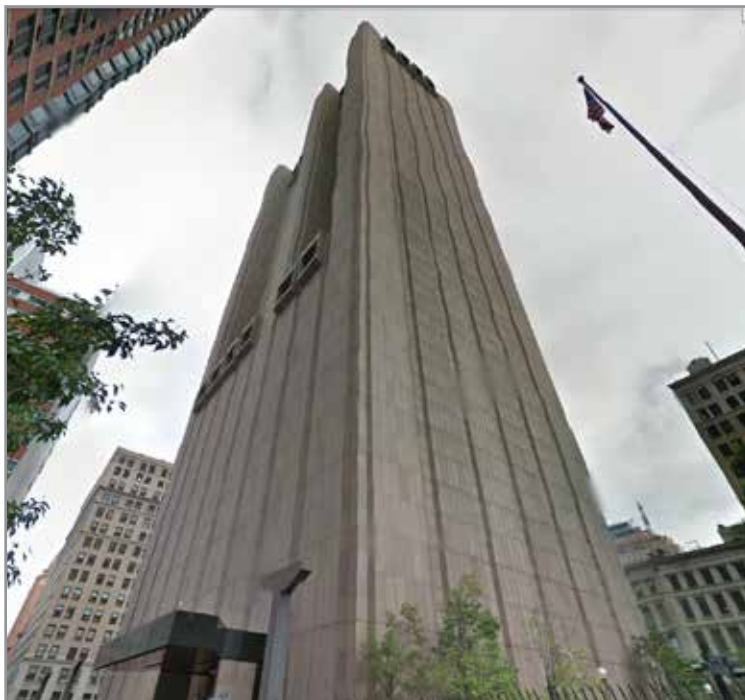
The former AT&T Long Lines building at 33 Thomas Street is one of a few major data centers and internet connection points in Manhattan that started out as telegraph or telephone company buildings. Photo from Google StreetView
