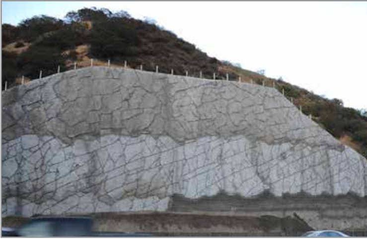
Stratigraphic detailing on the retaining walls of the 405 freeway.
