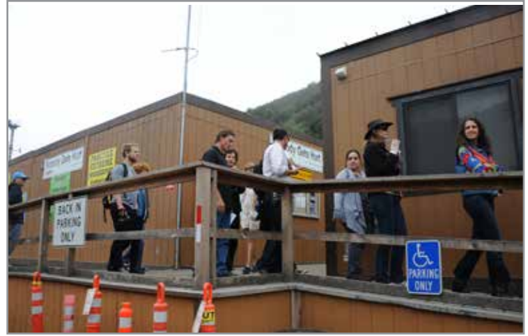
The group touring the office trailer compound at the Kiewit Yard in the Sepulveda Pass.
