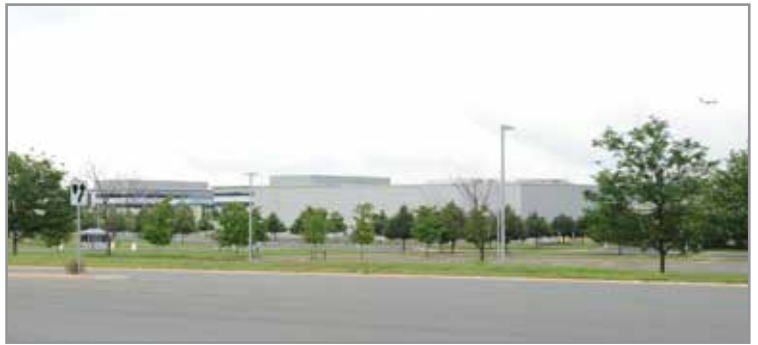
Verizon's Ashburn campus is where the telephone company and the internet meets the Federal government. The campus is located on UUNET Drive and was owned by MCI and WorldCom, before Verizon took over. CLUI photo
