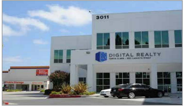
Digital Realty data center (next to an analog public storage facility) in Santa Clara, California, the biggest cluster of data centers in Silicon Valley. CLUI photo
