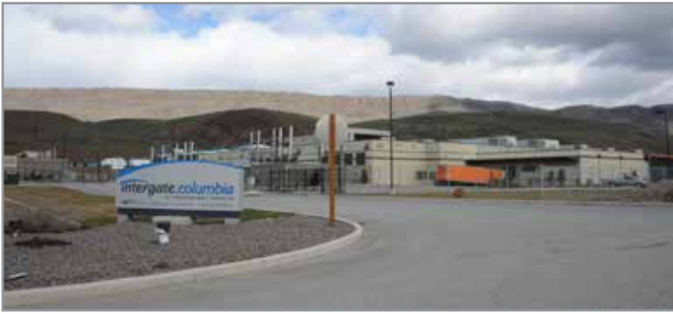
Further up the Columbia River, Sabey built a data center campus on a bluff in East Wenatchee, Washington. Phase one is complete, and leased out. Phase two will likely begin soon. CLUI photo
