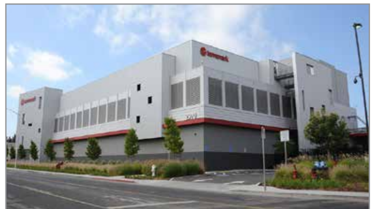
Terramark Data Center at 2970 Converse Street, in Santa Clara, California, one of the dozens of new data plants in the city. CLUI photo
